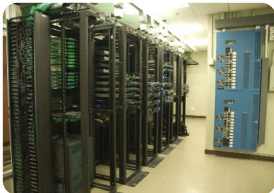
In the data center, *PANDUIT*® *DP6*™ *10Gig*™ Angled Patch Panels and *PATCHRUNNER*™ Vertical Cable Management work together to provide NASS with the highest density solution available.
